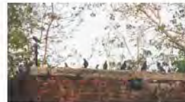
Building near overbridge with Rock Pigeons resting on it
