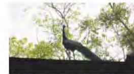
Peacock walks across the roof of the dilapidated mill
