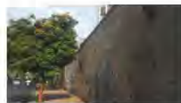
Mithakhali underbridge at one end of the track
