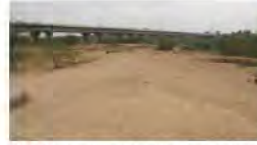
Dry river beds under the bridge
