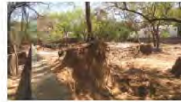
Open ground across the boundary wall
