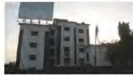
Multi-storeyed buildings along the railway track
