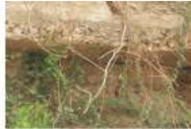
8. Salvadora persica has grown through the cracks of the P.C.C. slab. This plant has resistance to saline soils.
