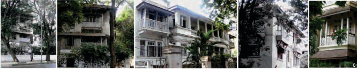
01 Porous building facade.
