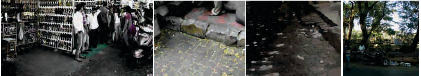
01 Encroached footpath, temporary stalls.
