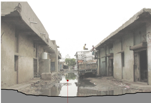
c. Stagnant & muddy water on internal road
