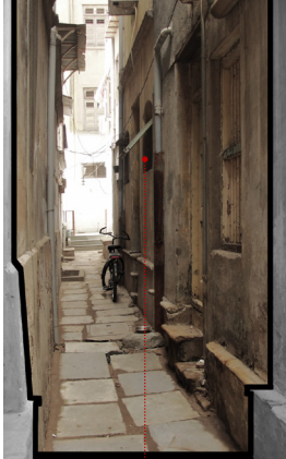
b Ventilation for toilets opens onto the narrow service lane between houses.
